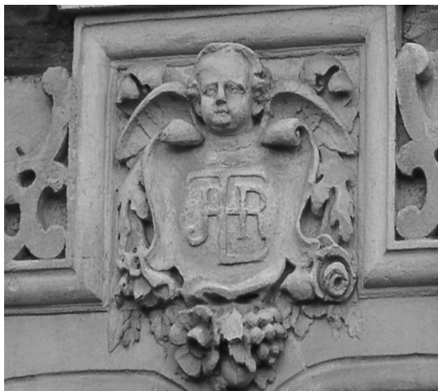
31 Trelawney Road. Door detail - the initials appear to be those of La Trobe
