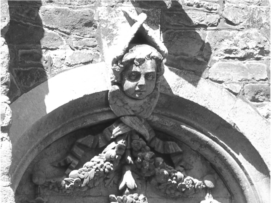
Detail of doorway, 33 Trelawney Road
