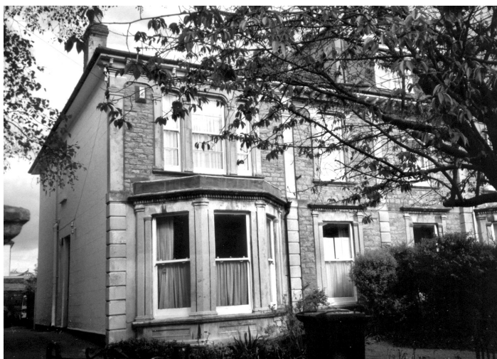
7 Elgin Park, showing the mixture of Bath stone and rubble stone on this side of the road.
