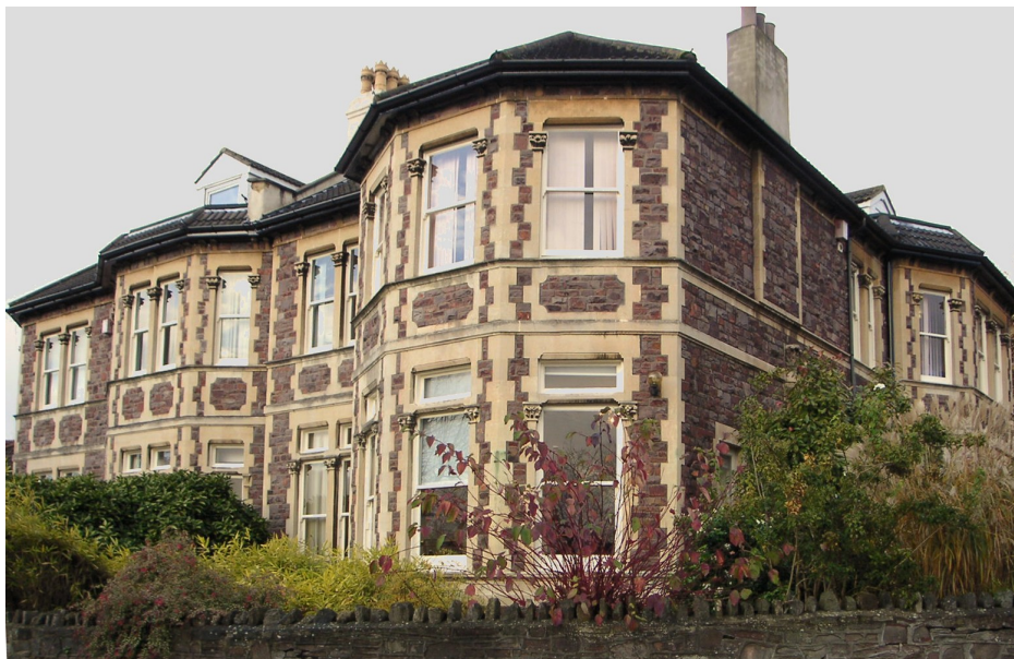
Above 7 and 9 Woodstock Road, originally Fairleigh and now part of the Redland High School
