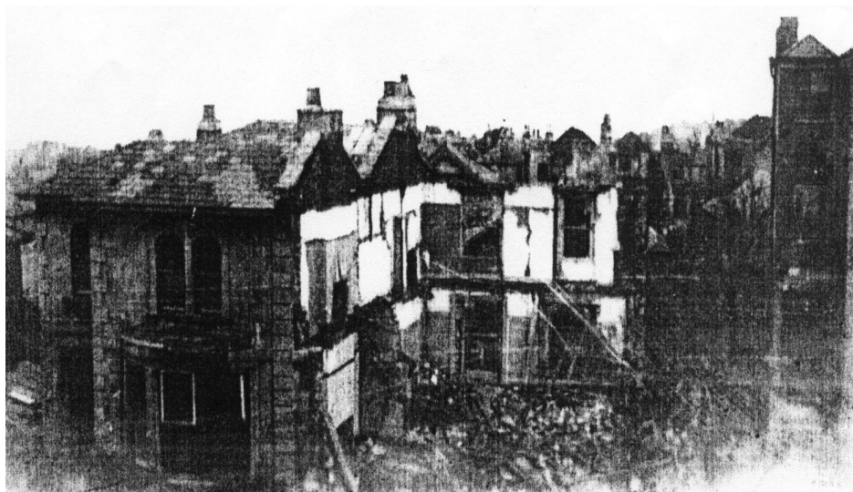
Above, bomb damage in Southfield Road.
